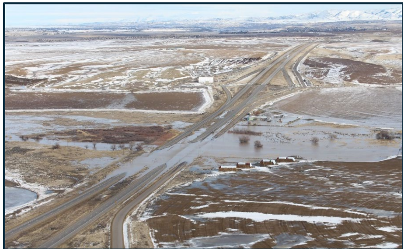
Figure 3: Raft River flood in 2017 over I-86.
