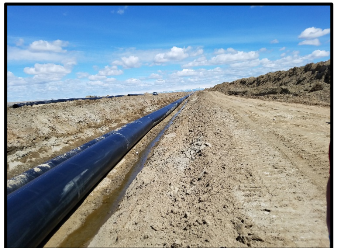
Photo 3 Farson Phase I Completed in 2016
